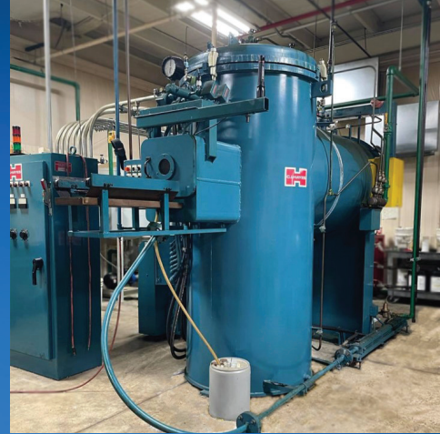
In-house Heat Treat Capability
